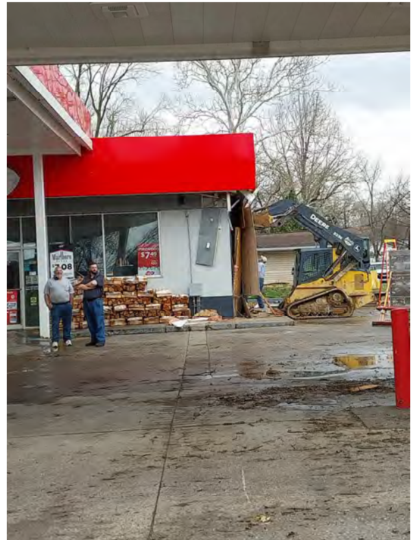
Left and right: the Oakland City On the Fly convenience store. Some windows are missing covered in plywood and the east wall is being supported by a bobcat.
